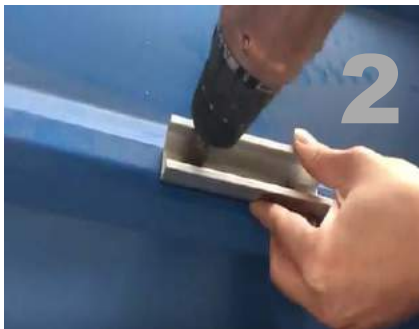
Fasten the mini rails with metal sheet roof with 2pcs of rubber pads and 2pcs st6.3*25 tapping screw.
